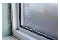
night follows a warmer day. Interior condensation forms on the inside of a window whenever there is excess humidity inside a home. It manifests in the form of condensation on the coldest areas of the wall — normally the windows. The warmer the air, the more moisture it will
