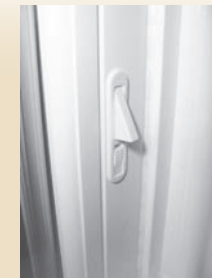
Vent latches are simply deployed and limit sash travel.
