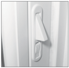
Vent latch, when deployed, will limit sash travel but allow for ventilation.
