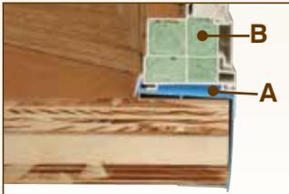
A. Exclusive welded sill pan (highlighted in blue) eliminates water penetration. The unique design provides a built-in weep system and a smooth finish on the exterior surface of the seat board.
